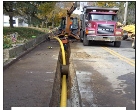
Roadway View: Typical Gas Main Pipe Installation
