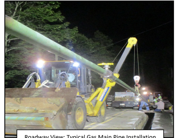
Roadway View: Typical Gas Main Pipe Installation
