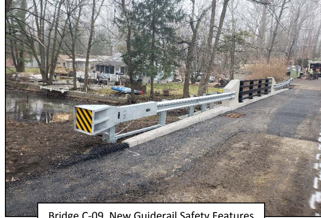
Bridge C-09, New Guiderail Safety Features
