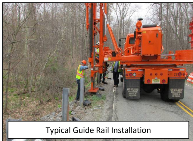
Typical Guide Rail Installation
