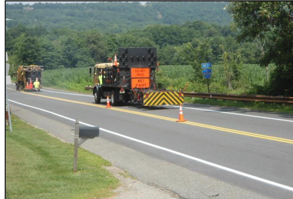
Typical Striping Operation
