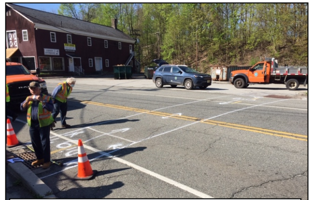
CR 631 Franklin Ave.: View of Project Site Looking West
