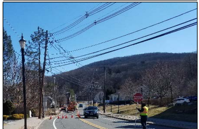
Typical single lane, flagger-controlled work zone setup
