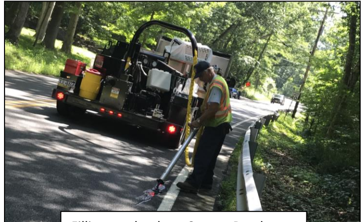
Filling cracks along County Roadways
