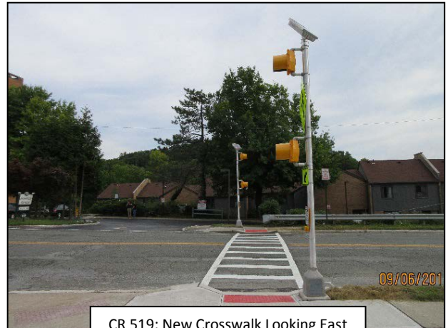
CR 519: New Crosswalk Looking East
