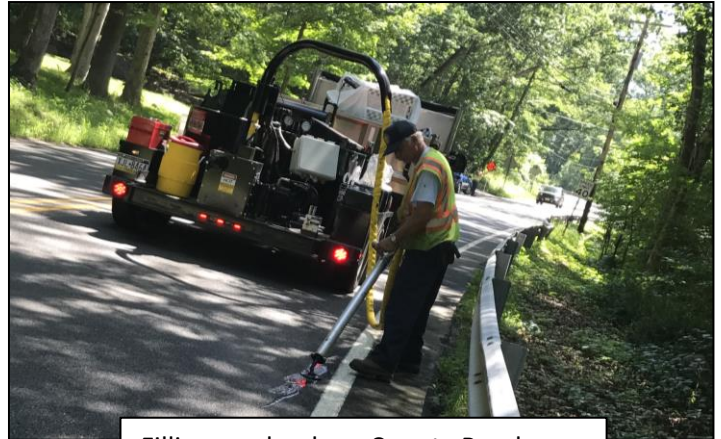
Filling cracks along County Roadways
