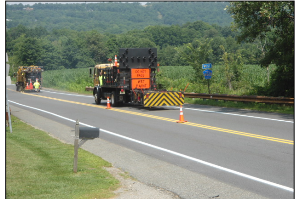
Typical Striping Operation
