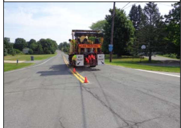
Typical Striping Operation
