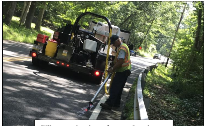
Filling cracks along County Roadways
