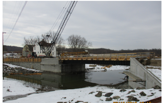
Deck & Retaining Wall Prepped for Concrete Placement
