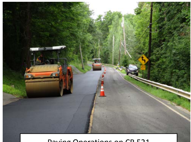
Paving Operations on CR 521
