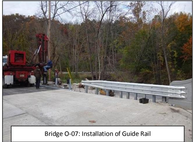
Bridge O-07: Installation of Guide Rail
