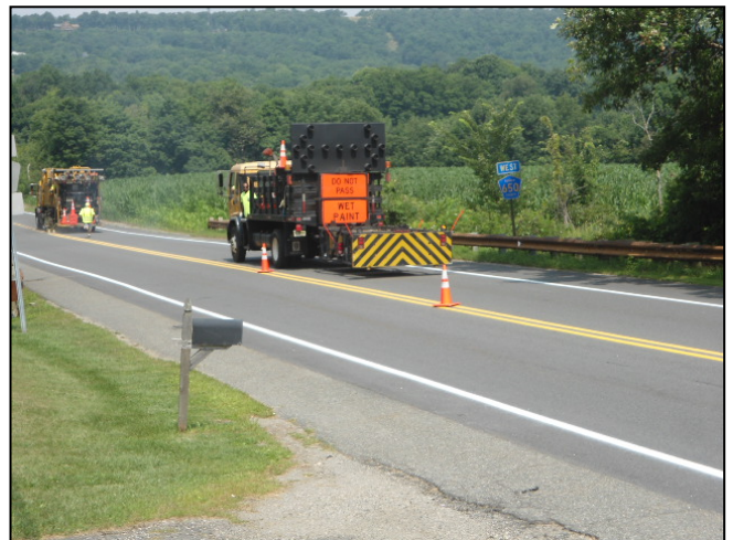
Typical Striping Operation
