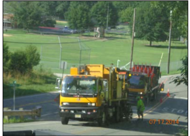
Typical Striping Operation
