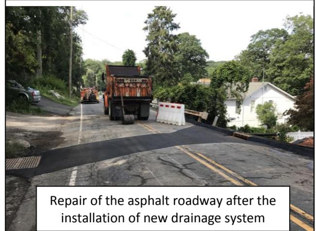
Repair of the asphalt roadway after the installation of new drainage system
