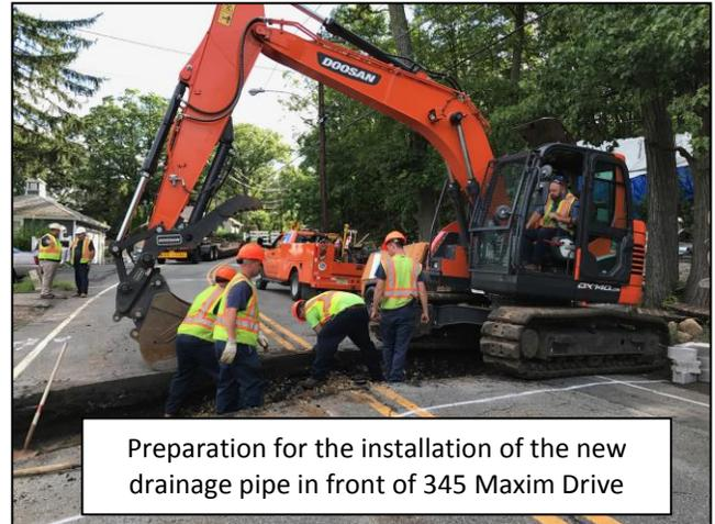
Preparation for the installation of the new drainage pipe in front of 345 Maxim Drive
