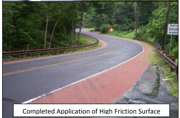
Typical High Friction Surface Operation
