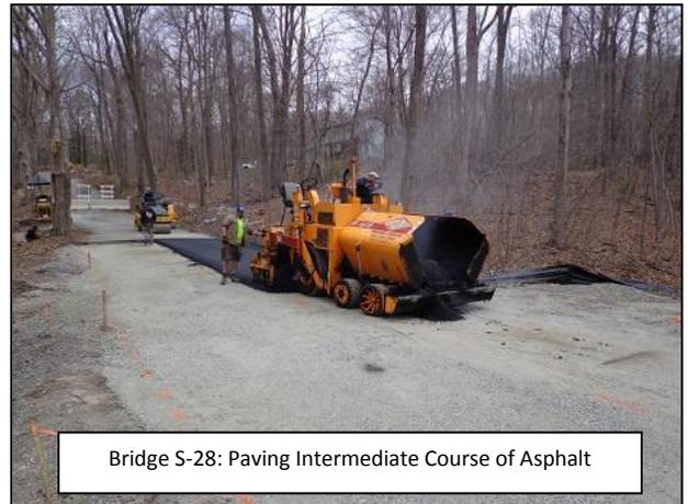
Bridge S-28: Paving Intermediate Course of Asphalt
