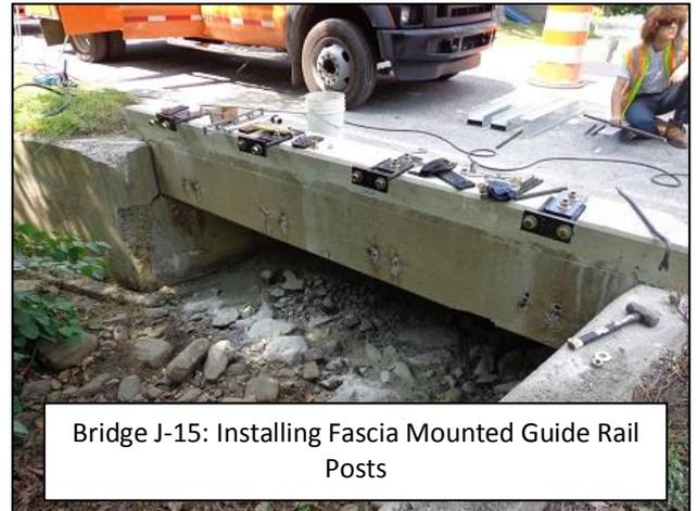
Bridge J-15: Installing Fascia Mounted Guide Rail Posts
