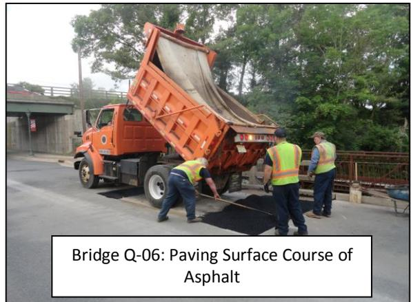
Bridge Q-06: Paving Surface Course of Asphalt
