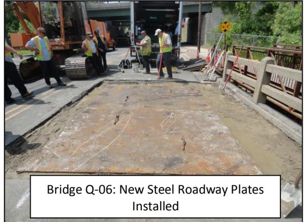
Bridge Q-06: New Steel Roadway Plates Installed
