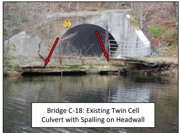
Bridge C-18: Existing Twin Cell Culvert with Spalling on Headwall
