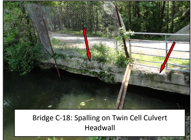
Bridge C-18: Spalling on Twin Cell Culvert Headwall
