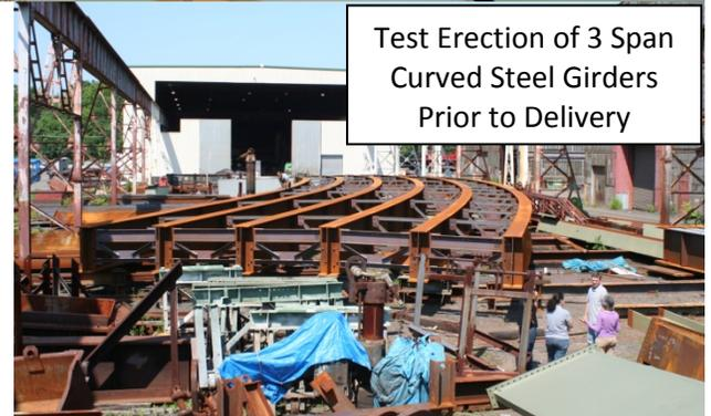
Test Erection of 3 Span Curved Steel Girders Prior to Delivery
