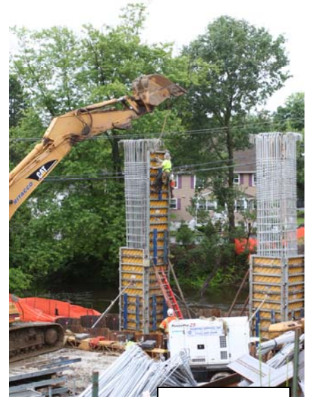
Closing formwork at Pier 1
