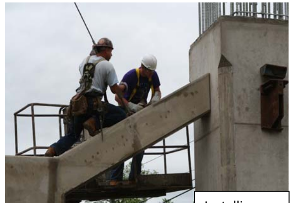
Installing Decorative X-brace
