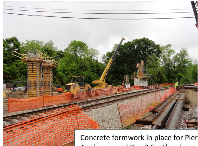
Concrete formwork in place for Pier 4 columns and Pier 3 South column
