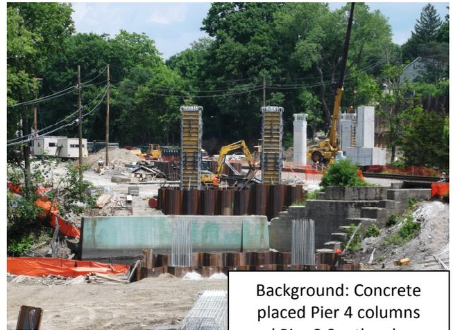
Background: Concrete placed Pier 4 columns and Pier 3 South column
