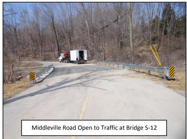
Installation of Guide Rail
