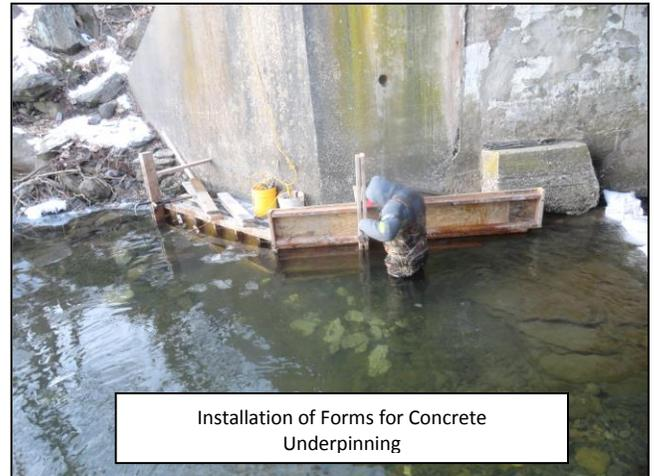
Installation of Forms for Concrete Underpinning
