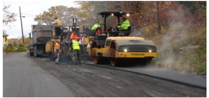
Typical Paving Operation
