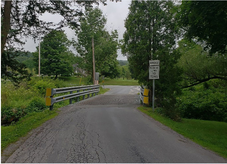
Bridge X-54: Approach Roadway
