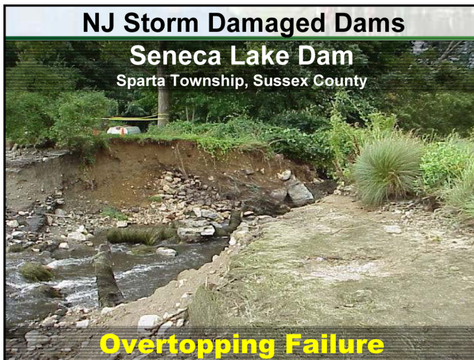
Figure 3.3.1-1: Seneca Lake Dam Failure Following Heavy Rainfall - August 12, 2000
