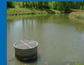
Detention Pond in North Carolina
