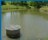
Detention Pond in North Carolina
