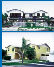
Top Picture: A house in Miami in the process of being elevated. Bottom Picture: That same house once completed. Taken from FEMA, Above the Flood, 2000
