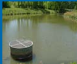
Detention Pond in North Carolina
