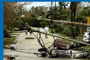
Fallen utility lines after Wilma. From www.galtmile.com
