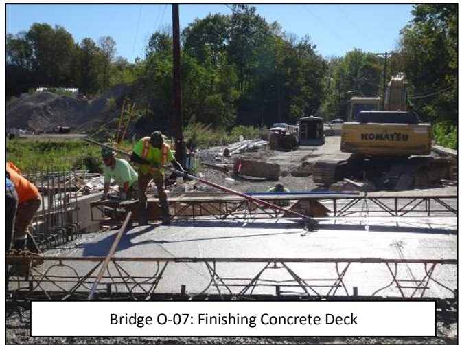
Bridge O-07: Installation of Concrete Deck
