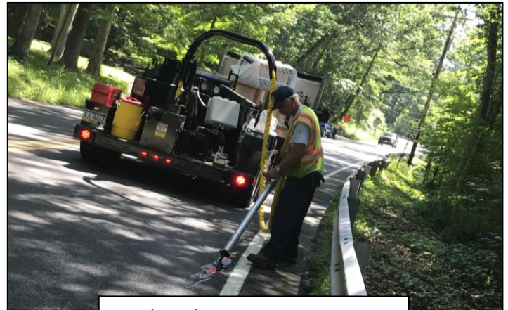
Crack Sealing Operations CR 607
