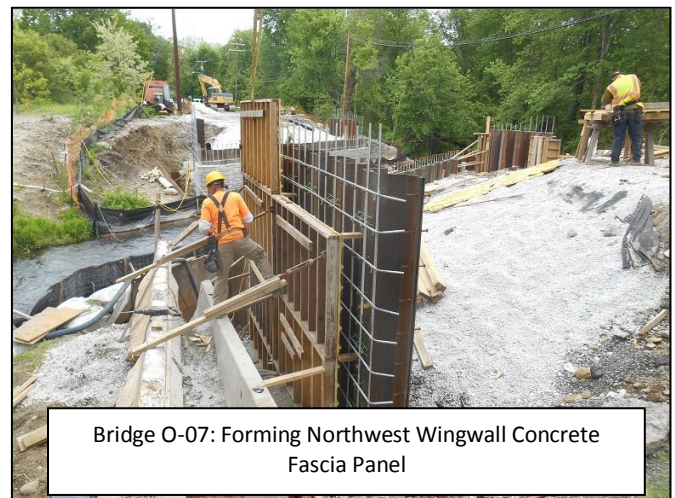
Bridge O-07: Tying Rebar for Wingwall Concrete Fascia Panel
