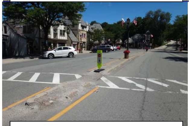
CR 613 Plaza Looking North
