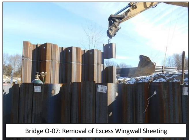
Bridge O-07: Removal of Excess Wingwall Sheeting
