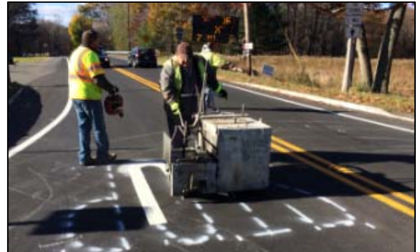
Traffic Marking Installation - CR 653
