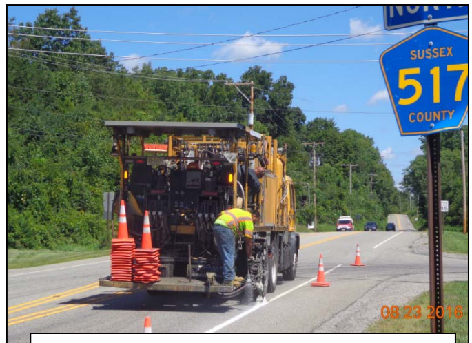
Epoxy Striping Operation - CR 517
