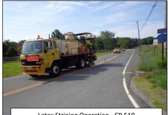
Latex Striping Operation - CR 519
