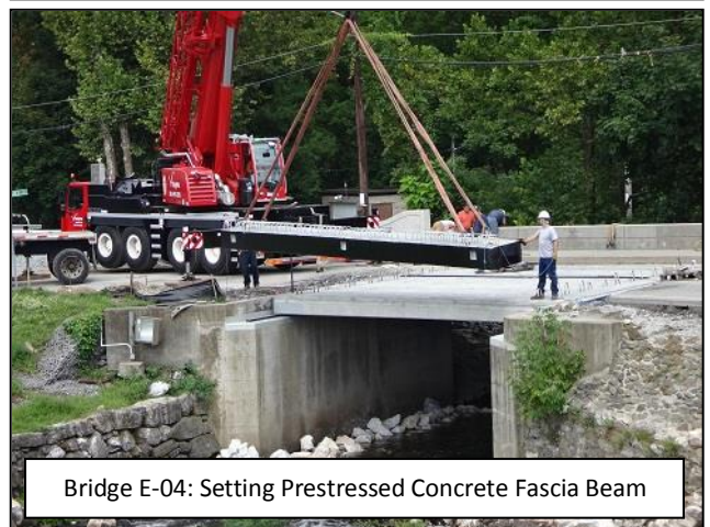
Bridge E-04: Setting Prestressed Concrete Beams
