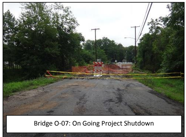
Bridge O-07: Current Road Closure
