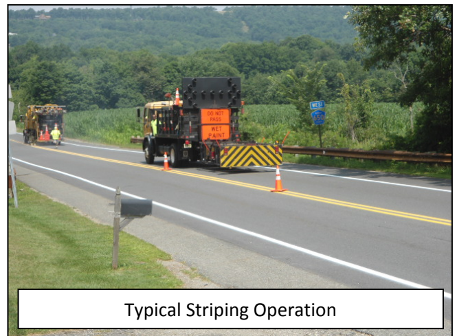
Typical Striping Operation
