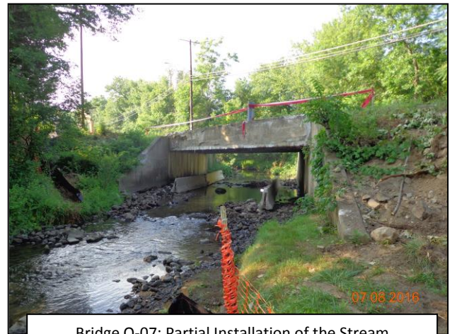
Bridge O-07: Partial Installation of the Stream Diversion
