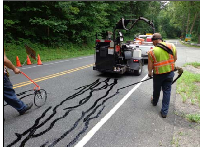
Typical Crack Sealing Operation
