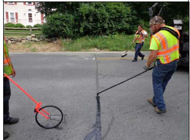
Typical Crack Sealing Operation
