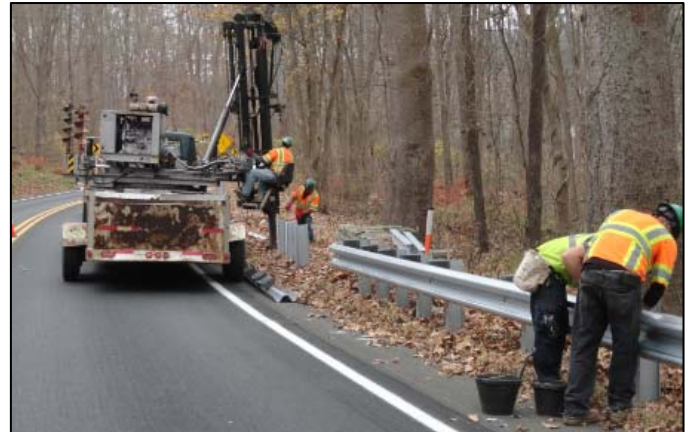
Guide Rail Upgrades – CR 560
