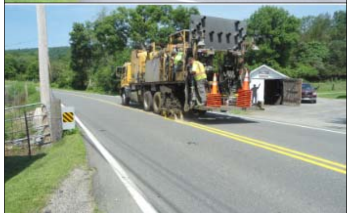
Typical Traffic Striping Operation
