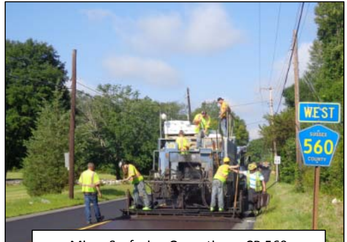
Micro Surfacing Operation – CR 560
