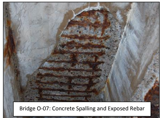
Bridge O-07: Bridge Fascia Deterioration Looking Downstream
