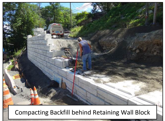
Installation of Precast Modular Wall Unit (Block)
