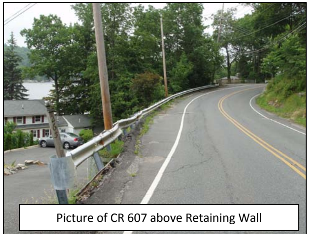
Picture of Existing Retaining Wall, CR 607 above.
