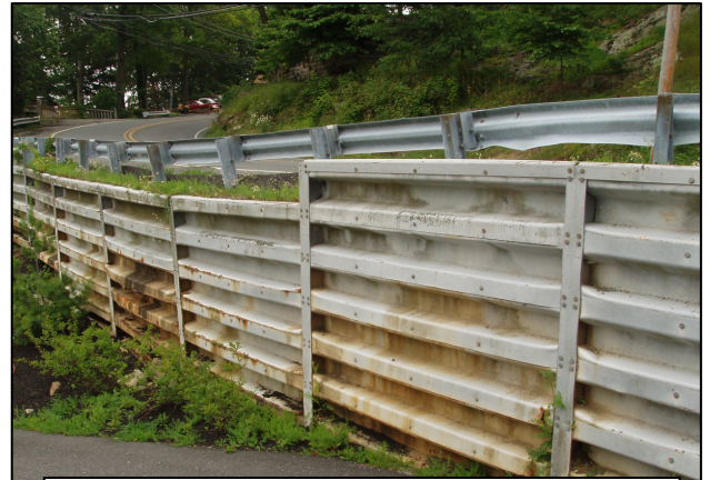
Picture of Existing Retaining Wall, CR 607 above.
